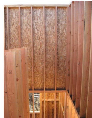
FIGURE 6 – FULL HEIGHT STUDS WITH BLOCKING AND NO PLATE BREAKS.
