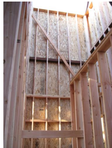
FIGURE 5 – FULL HEIGHT WALL STUDS WITH PLATE BREAK AND BLOCKING.
