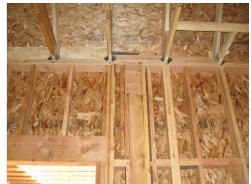
FIGURE 2 – H1 HURRICANE STRAPS INSTALLED ON THE INTERIOR FACE OF WALL.
