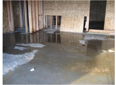
FIGURE 4 – WATER POOLING AT CENTER OF SLAB.
