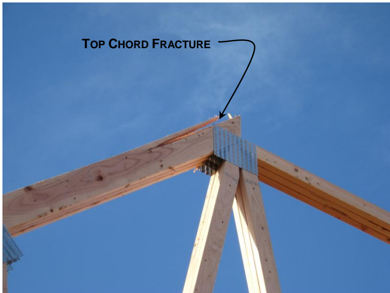
FIGURE 7 – PRE-MANUFACTURE WOOD ROOF TRUSSES WITH DAMAGE.
