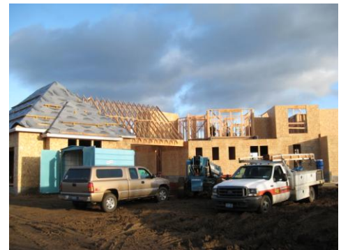
FIGURE 1 – PROGRESS OF STRUCTURE.
